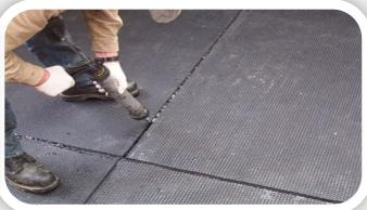
Quattro's range of high density mats can be bonded to new and existing floors using our Superflex Membrane The specially developed rubber adhesive achieves a strong bond to the rubber mats and subbase. Once the mats are in place the joints between the mats are cut out using a heated rubber groover. The cut strip is then removed to leave a clean open groove.
