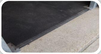
The joints are then sealed using our Q/Flex Gun applied flexible urethane resin as well as the perimeter of the area. Any residual sealant left on the surface of the mats will be removed with use.
