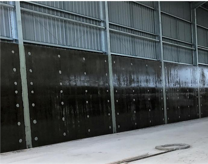
Q/seal is an air drying polyurethane pre-polymer with a high solids content and low viscosity for penetration into concrete floors/walls, grano or wood floors and walls. It exhibits excellent chemical resistance to a wide range of chemicals and first class abrasion resistance, is transparent brown in colour. It is recommended in areas subject to heavy wear, making it ideal for protection in some of the most aggressive environments.
