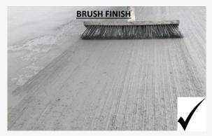
This is the perfect surface for our rubber to be fitted to as it is a flat level surface that provides a good key for our adhesives. Mats, pavers and tiles will sit flat and adhere well to the surface.
