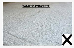
A Tamped Concrete finish is a ridged finish and is what we **DO NOT** want, as our rubber matting, pavers and tiles will not sit flat on to the concrete. The adhesive we use will sit in the low areas and will not bond the rubber. Joints of mats will also move when walked on. Unless it is a very low tamp we can not guarantee our flooring on this surface.
