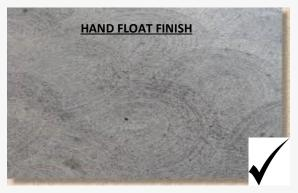
Hand Float finished concrete is good for fitting the rubber on to as long it is finished flat with no ridges in it.
