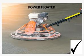
A Power Floated surface is a good surface for us to fit the rubber on to as long as it isn't finished very smooth like glass. If that was the case it may need scabbling to provide a key for materials like our Sportsroll.
