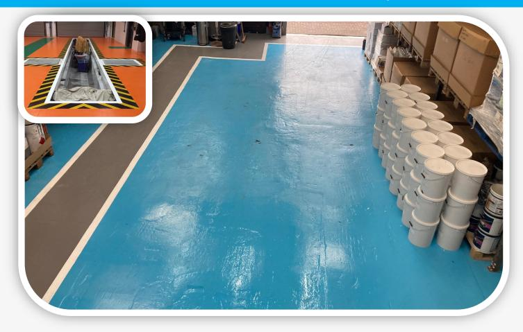
**Q/Shield SF** is a two-component 100% solids epoxy floor and wall coating offering excellent abrasion and chemical resistance. **Q/Shield SF** provides a tough, hard wearing coating giving high film build and wear resistance.
