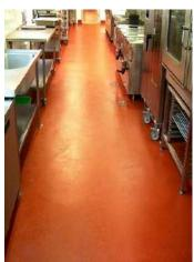
Heavy duty high build steam cleanable polyurethane floor
