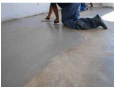
Floor Repair compound is a new concept for the repair of concrete and resin flooring. Floor repair is modified polyurethane concrete which has been specifically designed to provide an easy-to-use, primer free compound with exceptional physical properties. Floor Repair exhibits
