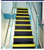
**Stair Treads & Stair Nosing** Made from orthophthalic resin and superior quality durable aluminium oxide grit.
